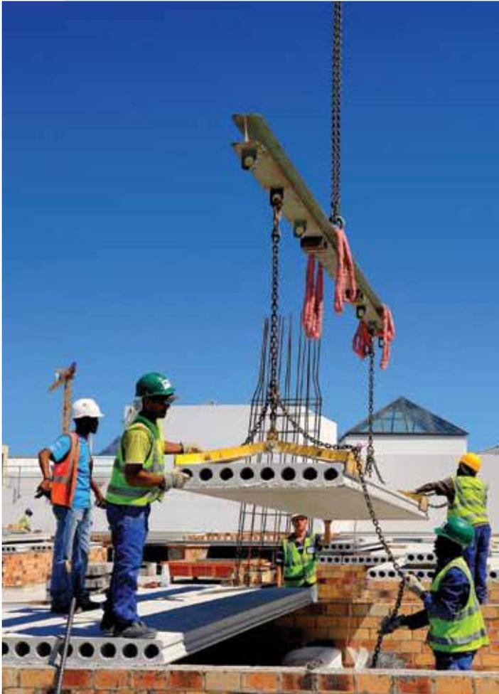
Because of the smaller size of the holes, formed in the slipform process, more concrete is needed per panel than needed when making use of extrusion. For the extrusion process this causes weight saving, reduces transport costs and causes the more efficient usage of the prestressing cable. The larger hole also makes it easier to accommodate service pipes conduits including down lights and transformers.
